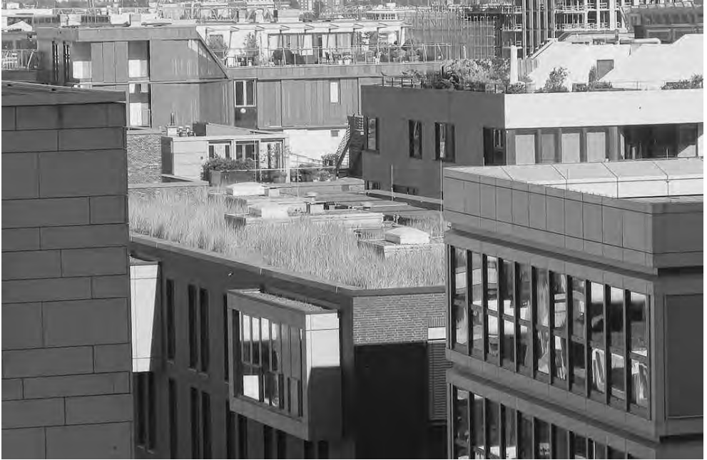
Fig. 4: Roofscape in Hamburg, HafenCity. Green roofs offer sites for vegetation without requiring additional space. Extreme conditions regarding climate, soil and water-supply pose challenges, to them vegetation technology has to find solutions. Photo: Westerholt, 2017
