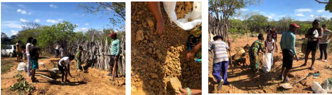
Figures 3-5 Group digging the clay pit and collecting the red clay
