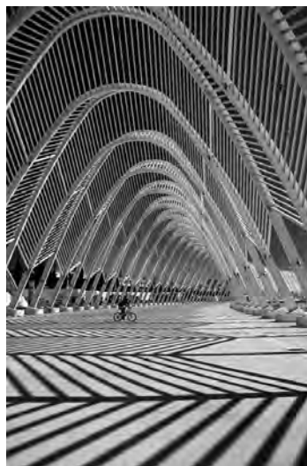
Fig. 8: OAKA Stadium in Athens. Photo by Yannis Prappas
