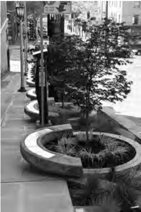
Fig. 14: Green Streets movement in Seattle. Storm water planters on Maynard green street by SvR Design Co.
