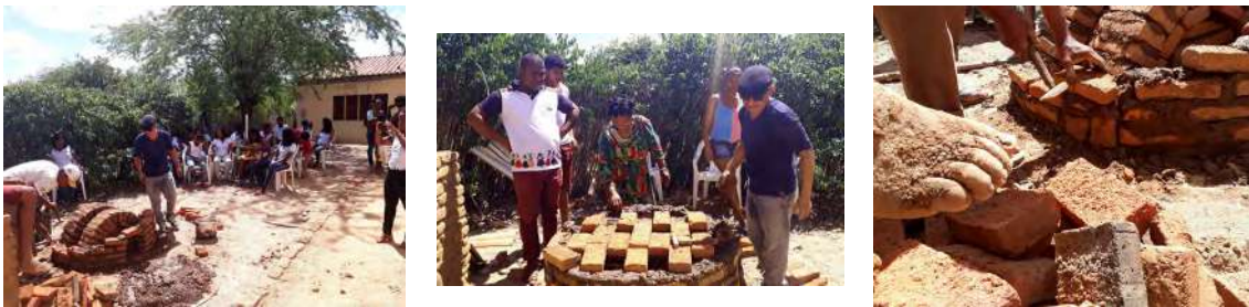
Figures 10-12 Oven building in progress
